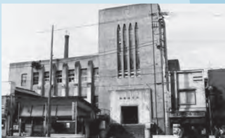
Denzuin Building, which was used as the head office at the time of our founding
